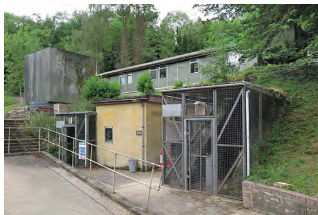
The main entrance to the Daws Hill bunker. The ‘dirty’ entrance is on the right. The ‘yellow’ building was codenamed ‘Sierra 2’ and was a fortified blockhouse for the security police. Photo Clive Penfold
